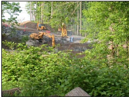
Figure 2. Small Construction Site
